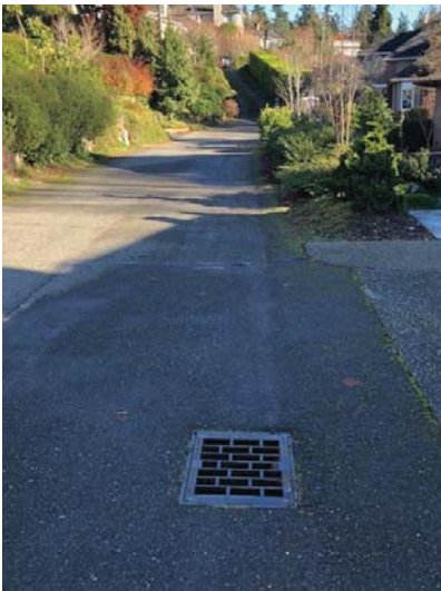
6 - Existing CB Downstream, Looking East.
