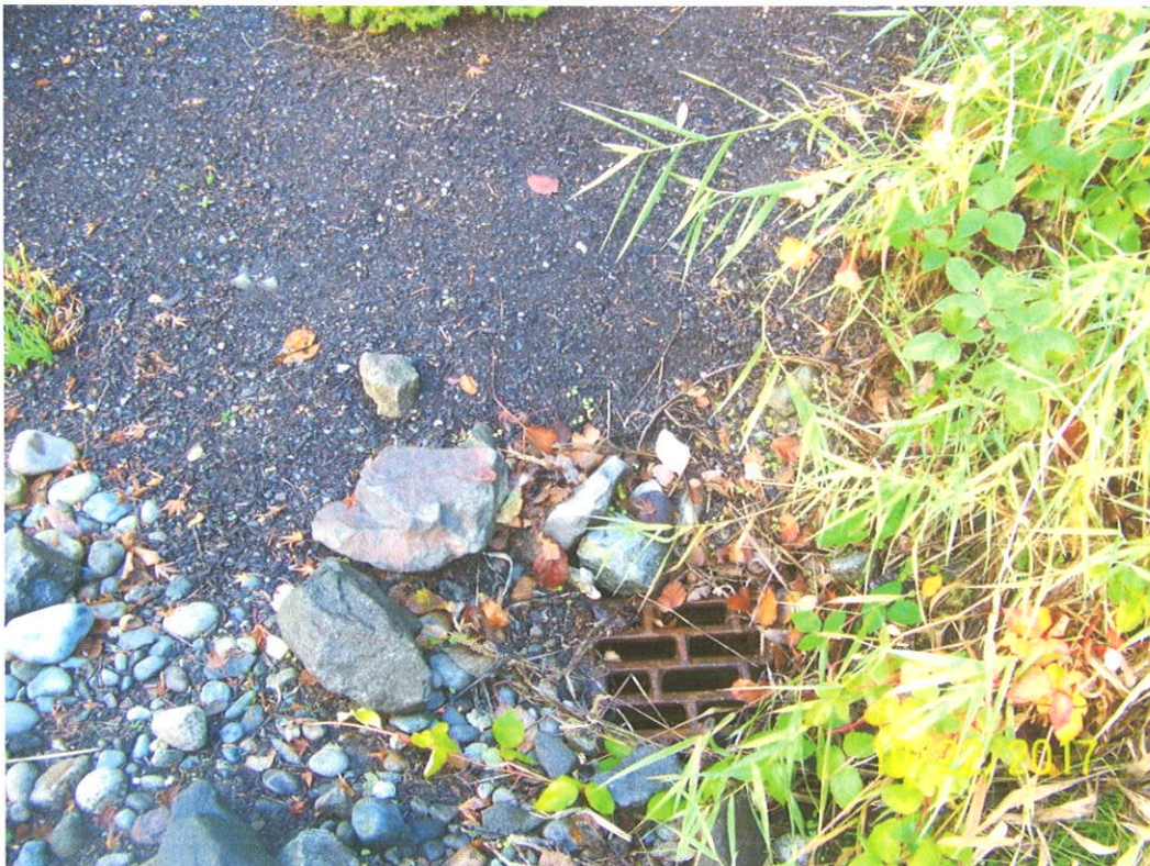
2) Storm drain at southeast corner of Property.
