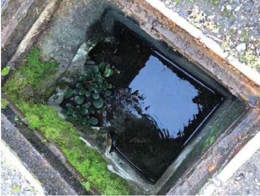
1 - Upstream Existing CB
