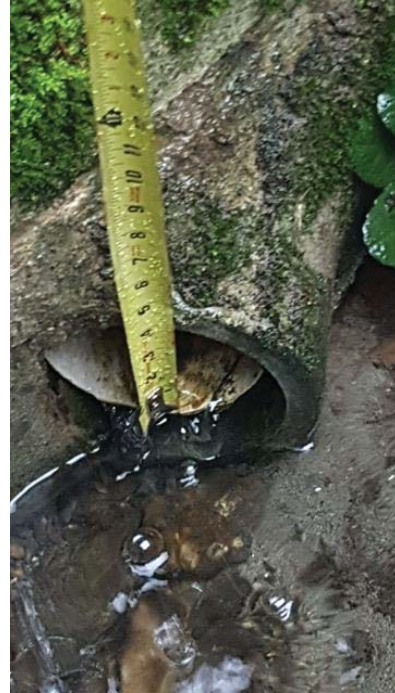
3 - Existing CB 4" PVC Inlet Rockery Wall Drain
